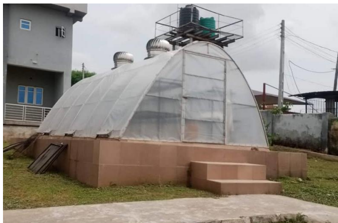
Fig. 1: NSPRI Parabolic Solar Dryer used for drying Cnidioscolus aconitifolius leaves.
